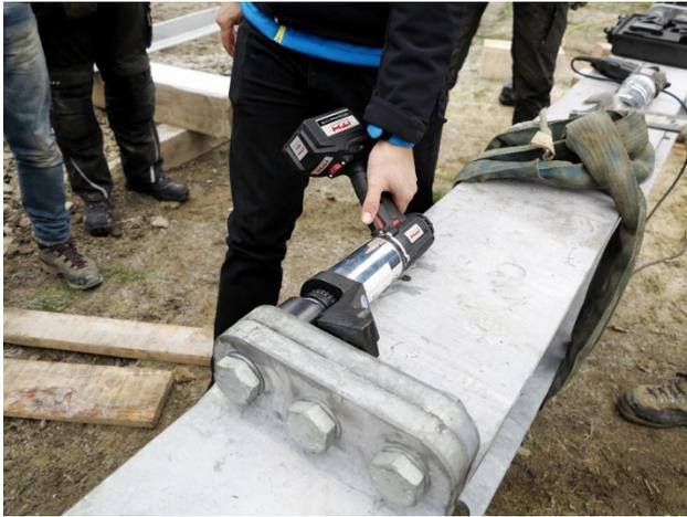
**Robust on-site design:** Battery nut runner ITH type ADS-150 tightens steel construction bolts of a cable railway.
