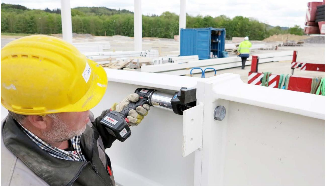
*By its newly designed and very compact gearbox the ITH nut runner type ADS is the battery torque wrench with the best power-to-weight ratio for torque ranges up to 4,000 Nm (2,950 ft\*lbs). In this picture the ADS-150 is shown tightening one HV-standard bolt connection size M27 (1 1/8") on an I-beam of [the new headquarter of ITH Bolting Technology](#) in Germany.*
